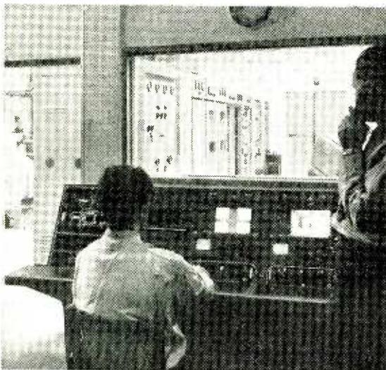
The control desk at the station, with the actual transmitter seen through the window.
